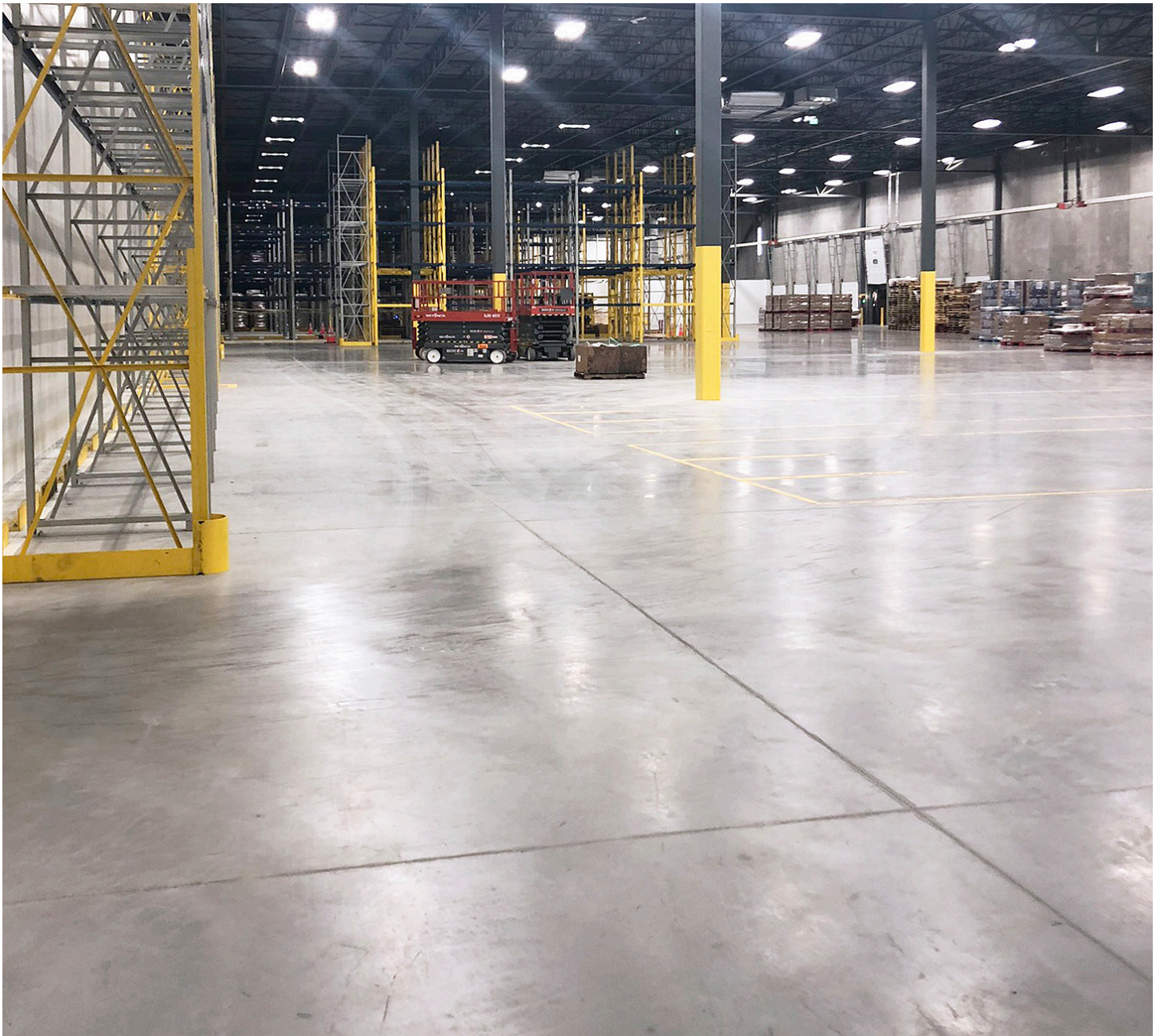
Fig. 2 Polished Warehouse Interior Concrete
