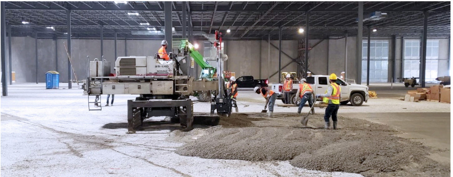
Fig. 8 Mars Industrial Canada Concrete Installation Somero installation with ground heating.
